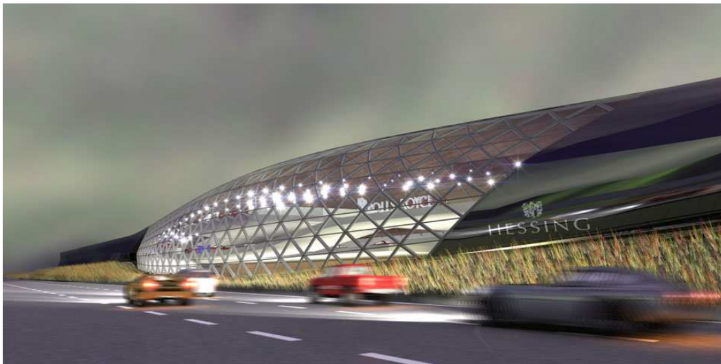
A2 Utrecht, the Cockpit: a showroom integrated in the noise screen
