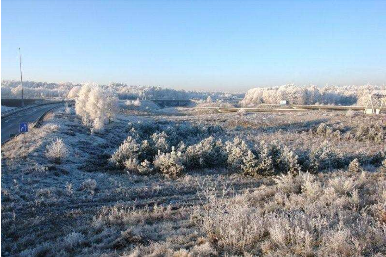
A12-A50 intersection Waterberg: because of the natural surrounding with fly-unders
