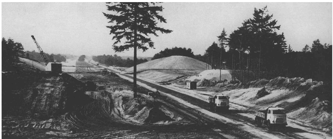
A28, cleaving the Veluwe, the largest forest area of the Netherlands
